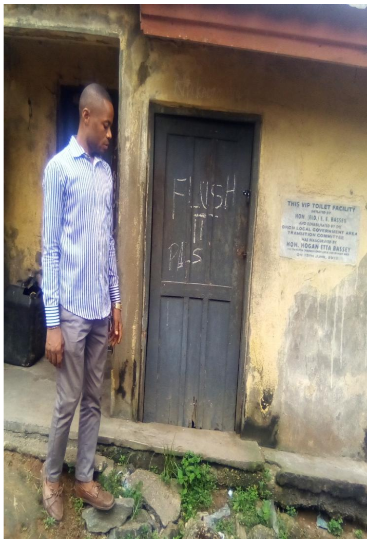
Plate 7: One of the researchers inspecting the public toilet facility in Uya Oro
